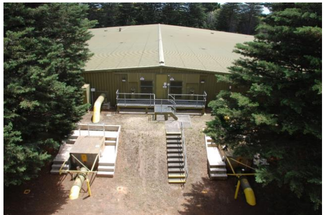
AERIAL VIEW OF THE KEW RESERVOIR Tony Michael, photographer, 2009
