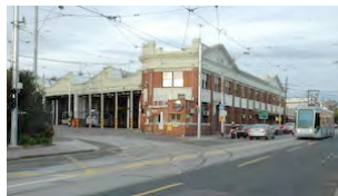
Kew Tram Depot, May 2008. Tony Michael, photograph
